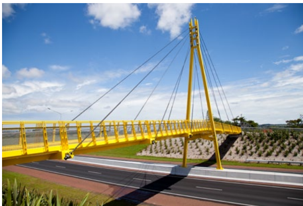
Motorway pedestrian bridge, Hobsonville.
