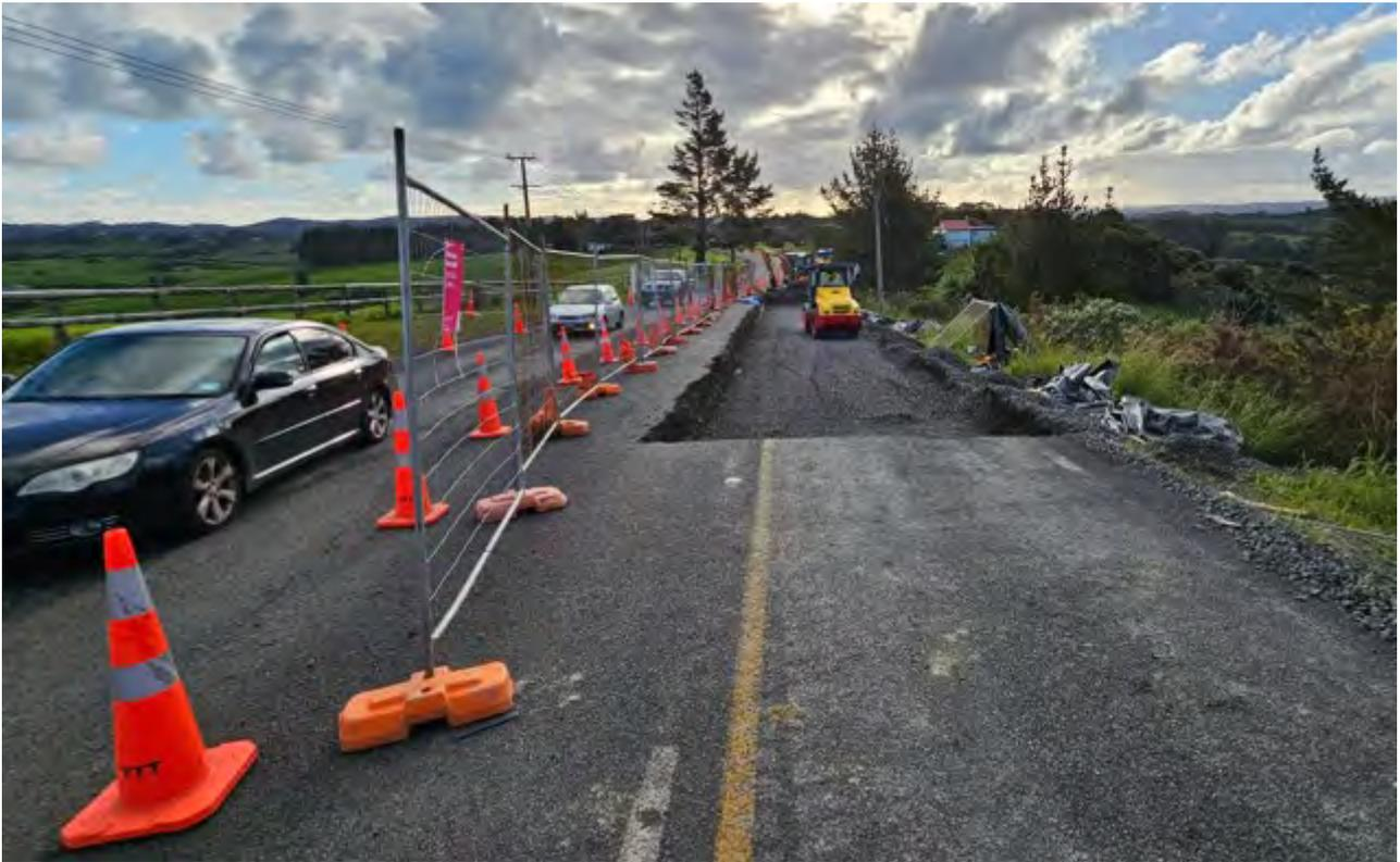
**780 West Coast Rd** Shoulder repairs and drainage work have been completed
