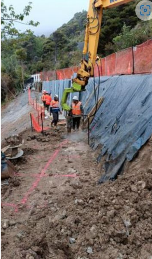
Piha road retaining wall under construction.
