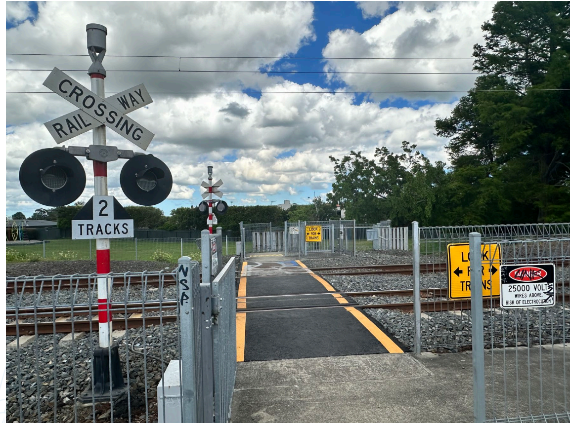
Automatic safety gates at Tironui Station Road East will be reused as an interim safety improvement at O'Neills Road.
