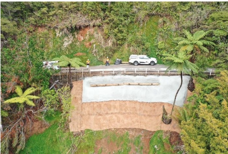
Slip repairs on Karekare Road
