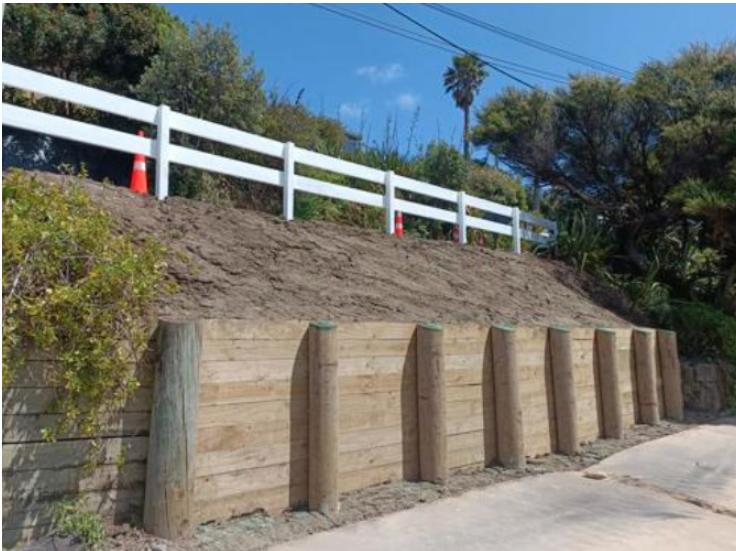
Repairs at 27 Rayner Road
