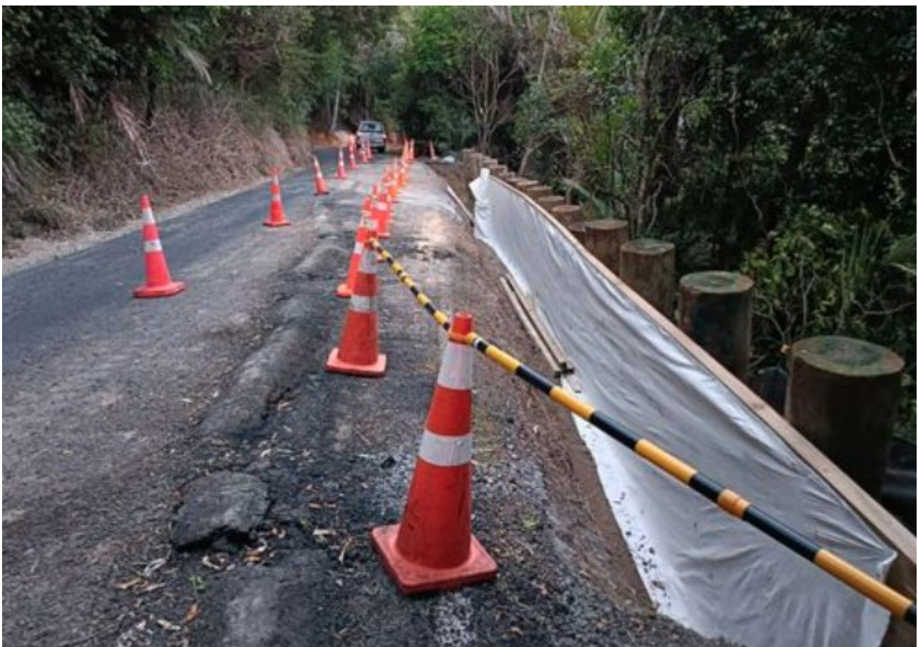
Titirangi Beach Road repairs underway
