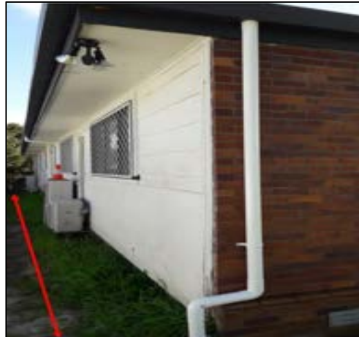
New downpipe installed
