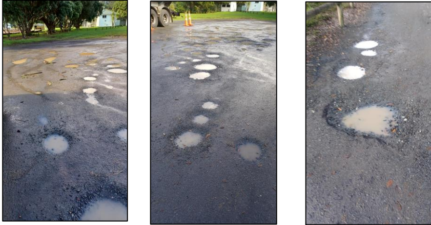
Before remedial work completed
