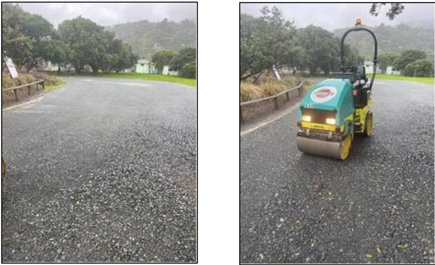
After remedial work completed
