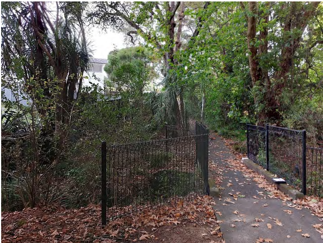
Picture 2 – Culvert crossing at Glen Eden Picnic Ground
