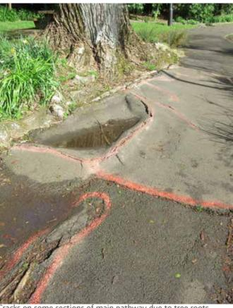
Cracks on some sections of main pathway due to tree roots
