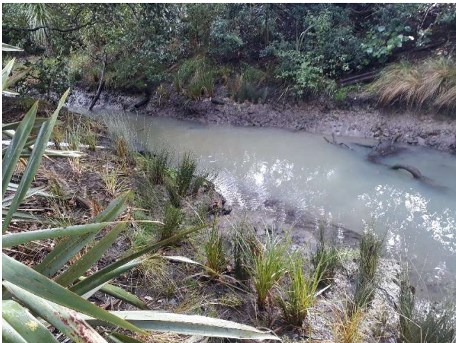
Photo: Finished bank planting at Rothesay Bay
