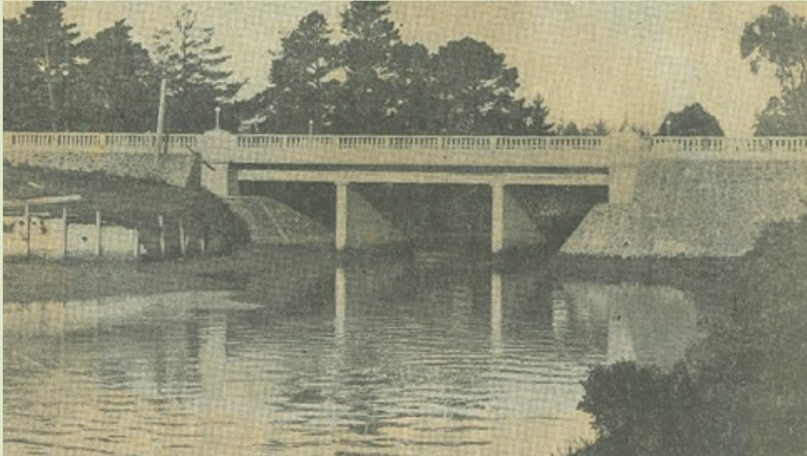
The new reinforced concrete Whau Bridge, July 1932 (Auckland City Council Works Department classified subject file on the Whau Bridge, 1920-1956, Auckland Council Archives, ACC 219/380b)
