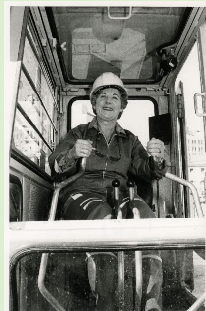
Ground-breaking ceremony for Aotea Centre with Mayor Tizard driving the digger, 5 August 1985 [Auckland City Council Photographic Department, Auckland Council Archives, ACC 497/3bs]
