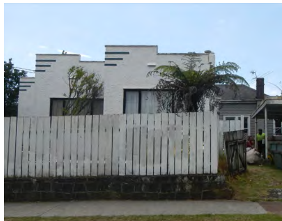
Art Deco style, Mars Avenue (non-contributor because built after 1940)
