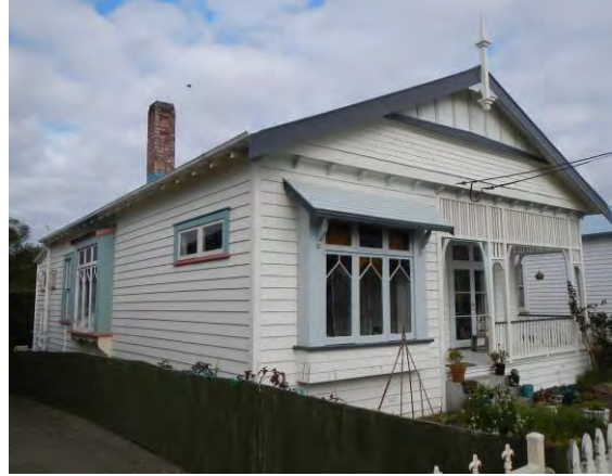
Transitional villa, Halston Road
