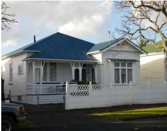
Transitional villa, Halston Road
