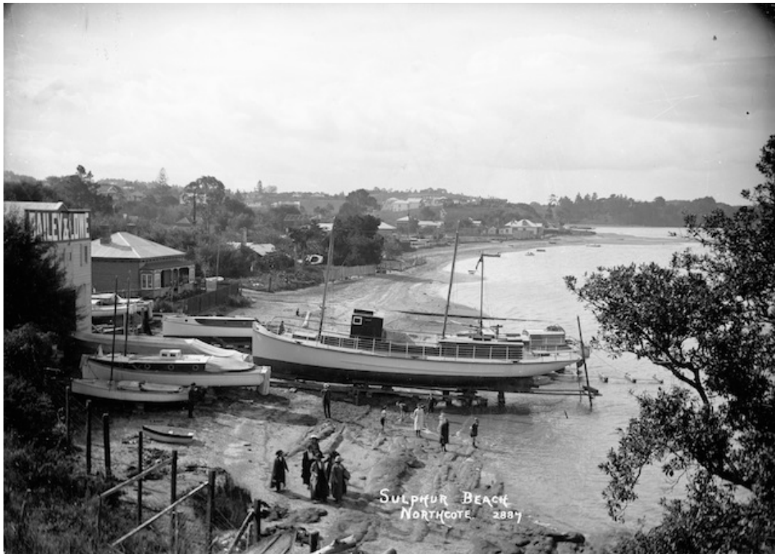
Fig. 40. Bailey and Lowe boatshed and slipway at Sulphur Beach, Northcote, 1913. The Lady Eva is shown on a cradle at the centre of the image. Photographer: William Arthur Price, Alexander Turnbull Library, Wellington, N.Z., C-1690-1/2.
