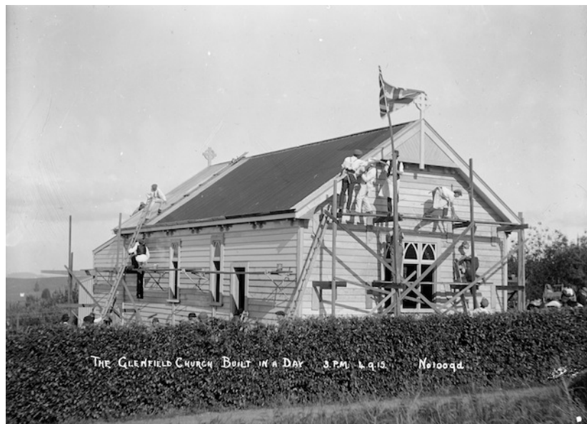
Fig. 61. Some buildings served as churches for a number of denominations. The Glenfield Mission Hall was built to by the local community in a single day and it is shown here almost complete at 3pm on 4 September 1915. Anglican, Presbyterian and Methodist services were held on successive Sundays in the hall and it also served a number of other community purposes. Alexander Turnbull Library, Wellington, N.Z., G-1862-1/2.
