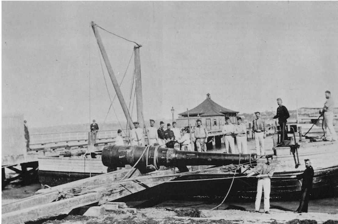
Fig. 52. Thirteen-ton cannon being unloaded from a barge at Victoria Wharf for installation on Mt Victoria in 1899. Auckland War Memorial Museum, C16566.
