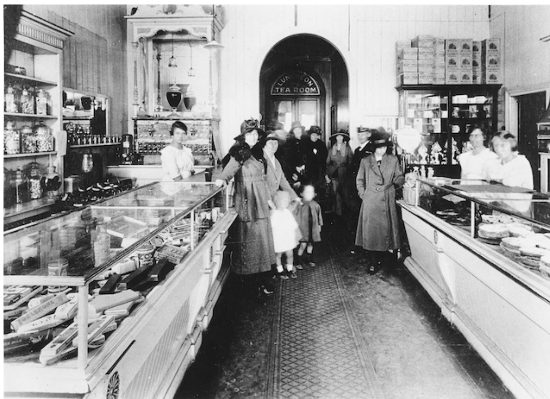
Fig. 42. Interior of E. Ford's Irresistible Tearooms in Victoria Road, Devonport, 1925. North Shore City Libraries, D_PB_0002.
