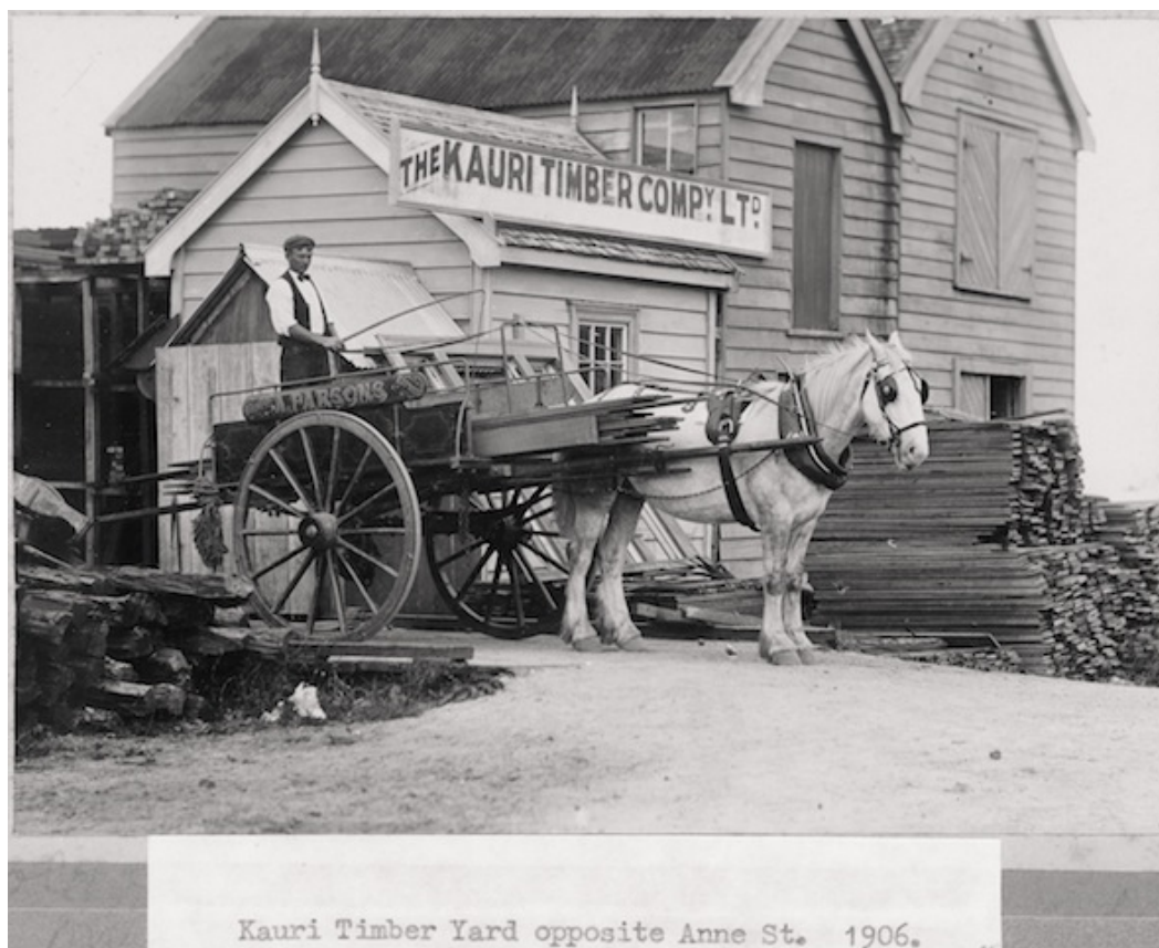
Fig. 36. Kauri Timber Company Limited, Devonport, 1906. North Shore Libraries, D_GBB_0006.
