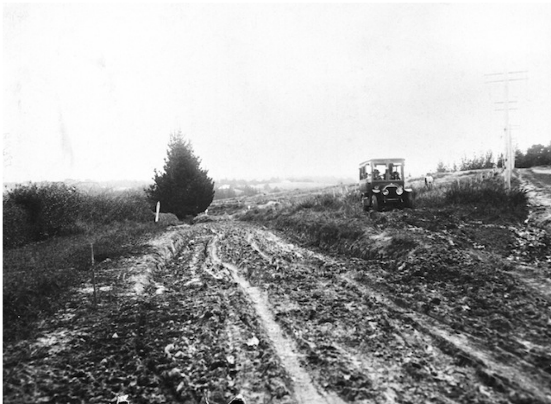
Fig. 10. Roads were sometimes in very poor condition, particularly in winter as this image taken in 1926 at the corner of Glenfield and High Roads shows. The driver of the Birkenhead Transport Company bus found the bank alongside the road easier to negotiate than the road itself. Sir George Grey Special Collections, Auckland City Libraries, 7-A11043.
