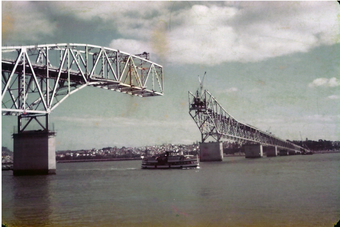
The MV Albatross sails beneath the almost complete Auckland Harbour Bridge, 1958. PHG LaVie © Elizabeth Lancaster, North Shore Libraries, N0116015
