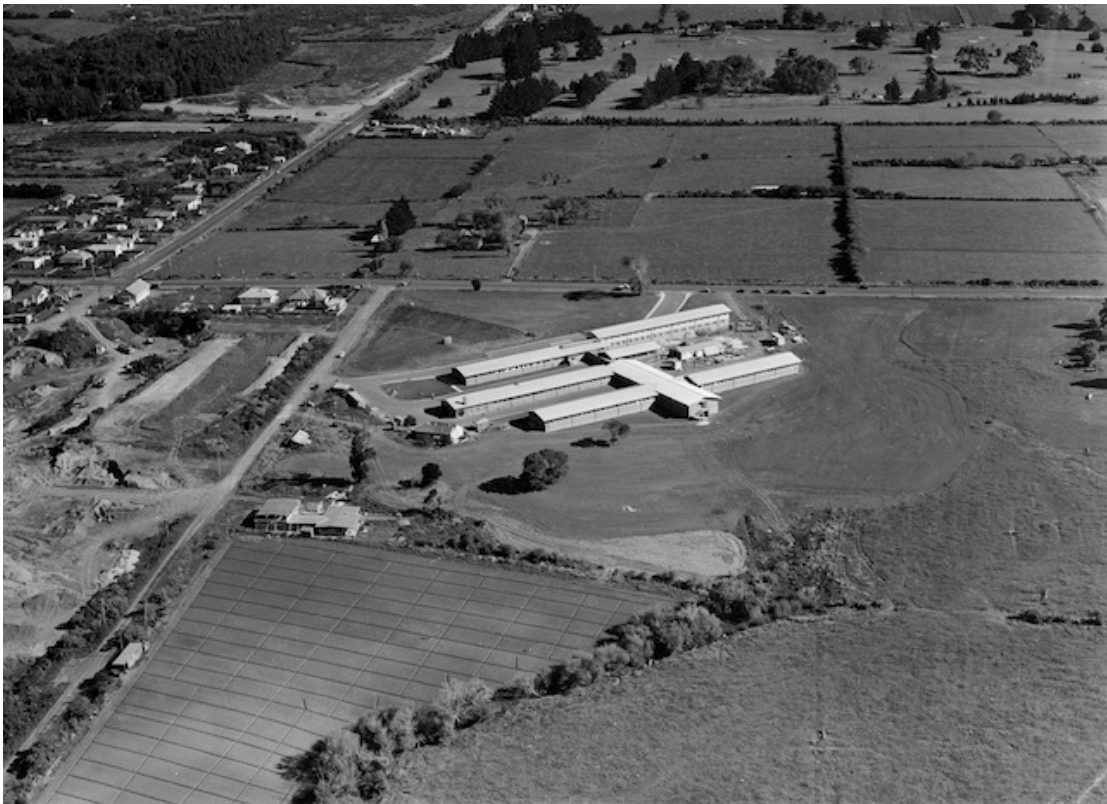
Fig. 59. Aerial view of North Shore Hospital under construction in April 1958. Whites Aviation Collection, Alexander Turnbull Library, Wellington, N.Z., WA-43637.
