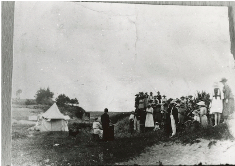
Fig. 60. The absence of a local church did not prevent services from taking place. This outdoor church service was held at Mairangi Bay in 1923. North Shore Libraries, T2304.
