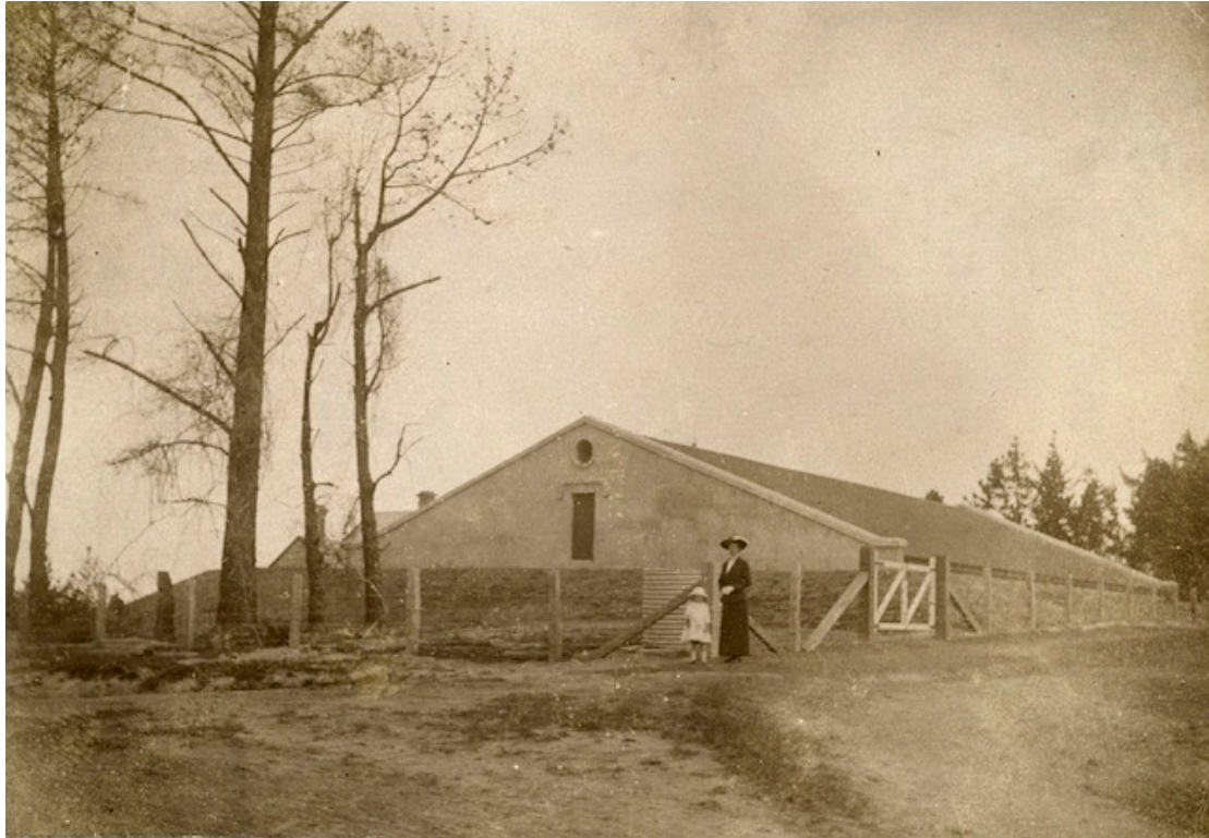
Fig. 16. This reservoir in Waipa Street, Birkenhead held water pumped from Lake Pupuke. North Shore Libraries, B0325.
