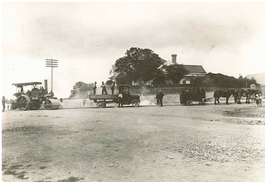
Fig. 11. Roadmaking was an expensive and labour intensive undertaking as shown in this image of road improvements at the corner of Mokoia and Rawene Roads. North Shore Libraries, B0310.
