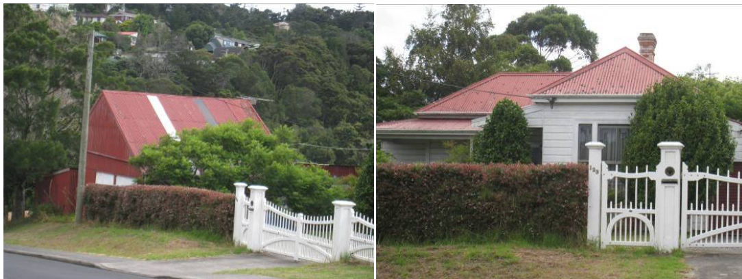
Fig. 6 [left] & Fig. 7 [right] Cox's barn at 123 Stanley Road Glenfield is a rare example of a surviving farm building. It is scheduled Heritage inventory no. 29. Cox's house is also scheduled. Photo Matthews and Matthews Architects Ltd, 2010.
