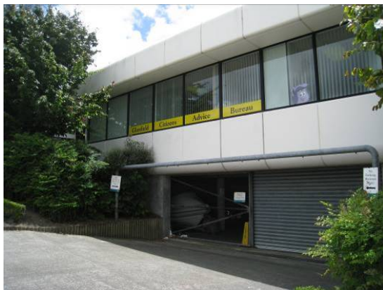
Fig. 9. Council's Glenfield District Office in Bentley Avenue. Photo Matthews and Matthews Architects Ltd, 2010.
