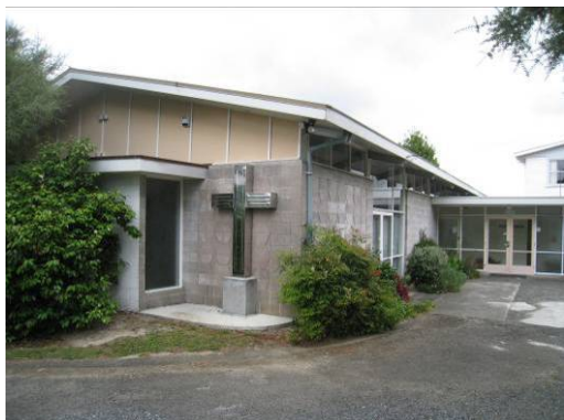
Fig. 13. St Barnabas Anglican Church at 470 Glenfield Road. Photo Matthews and Matthews Architects Ltd, 2010
