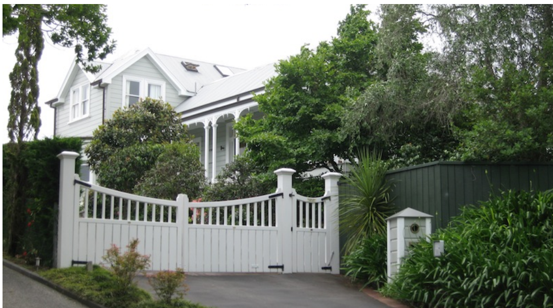
Fig. 4. Cave house, View Road. Photo Archifact.
