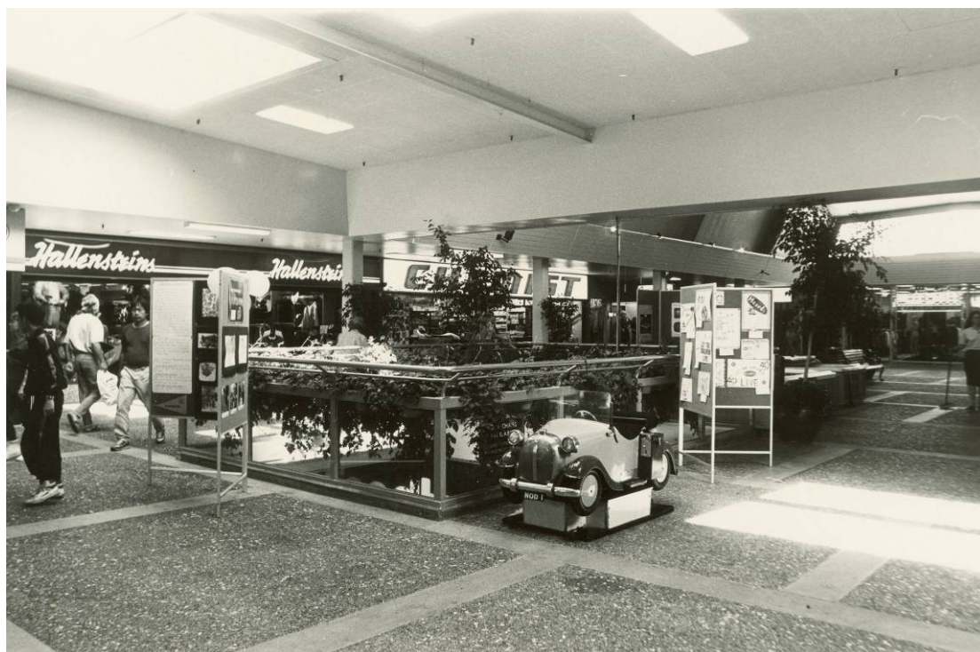
Fig. 8. Upper floor inside Glenfield Mall, 1990. North Shore Libraries, T1813.
