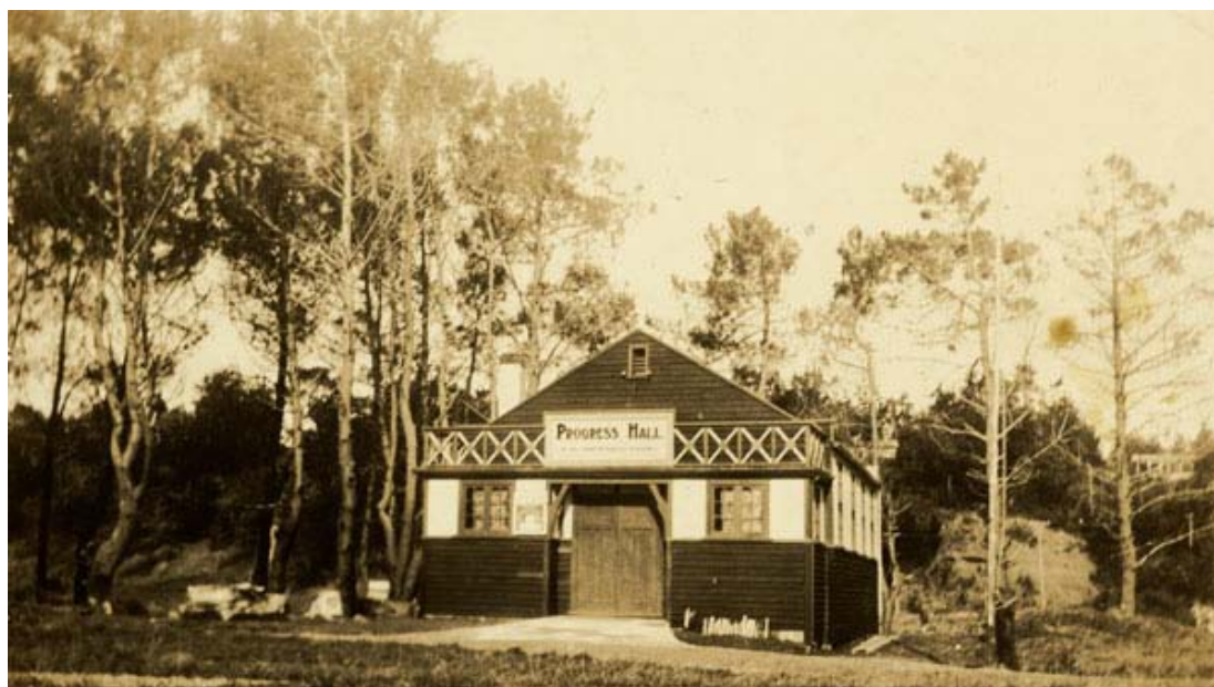
Fig. 15. Progress Hall, Anzac Road, Brown's Bay. North Shore Libraries, E0341.
