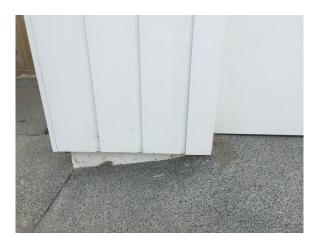
E2/AS1 compliant ground clearance at garage door
