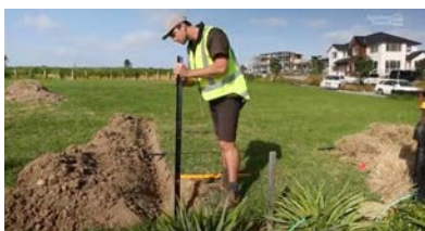
Building a silt fence and bunds 4:57
