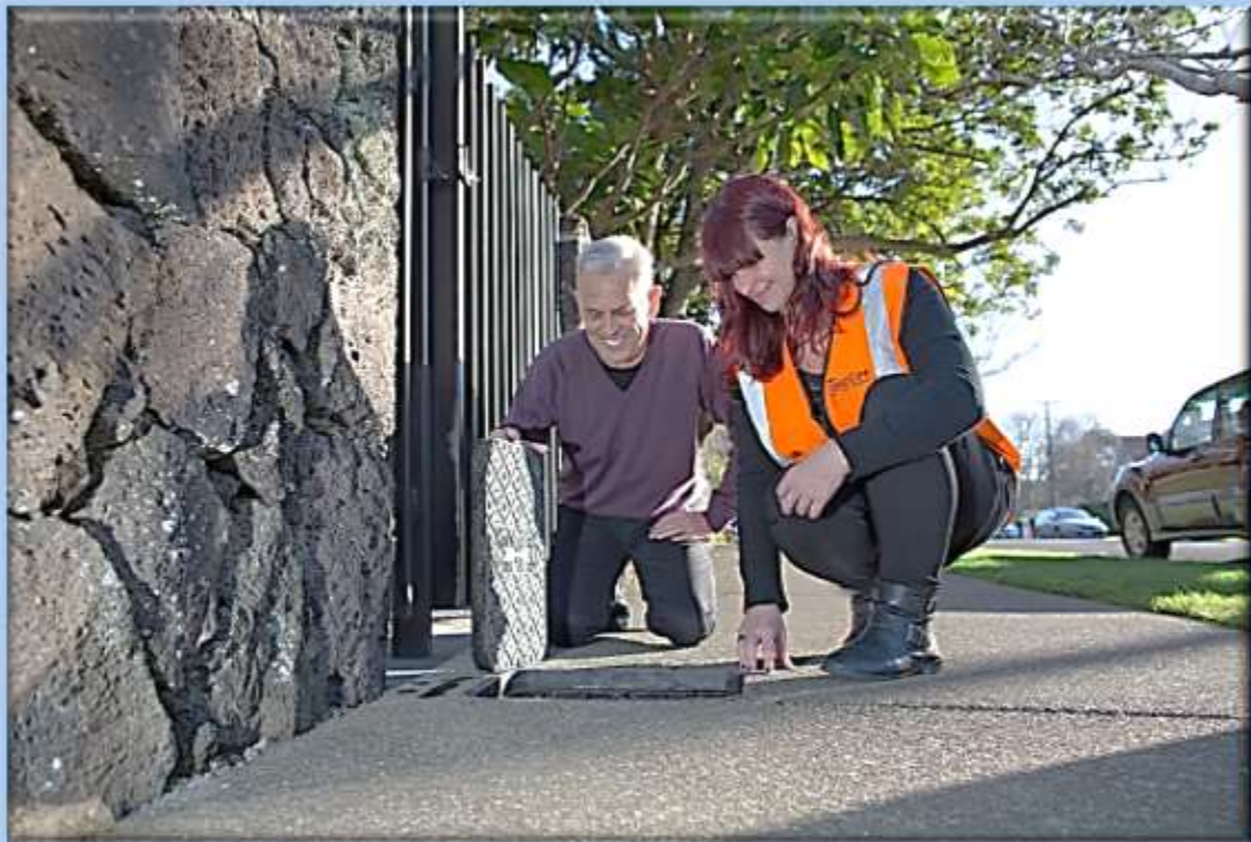
Leanne McKenzie, Water Quality and Compliance Analyst, demonstrating how to conduct a leak test.
