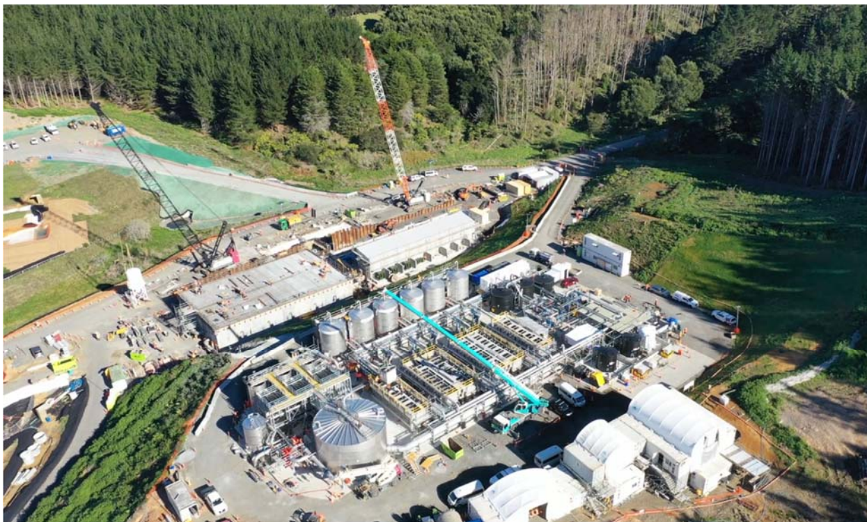
Our newly completed Waikato 50 water treatment plant
