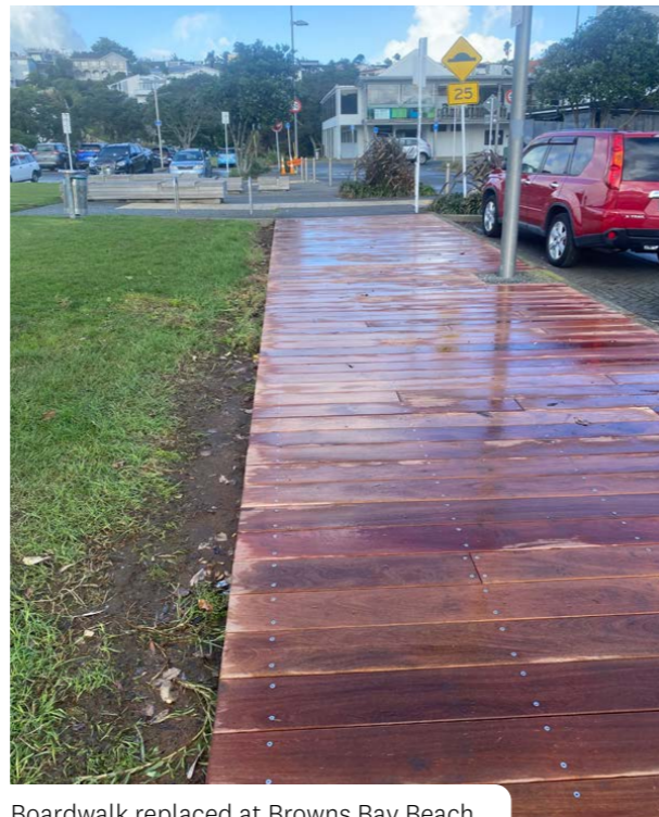
Boardwalk replaced at Browns Bay Beach
