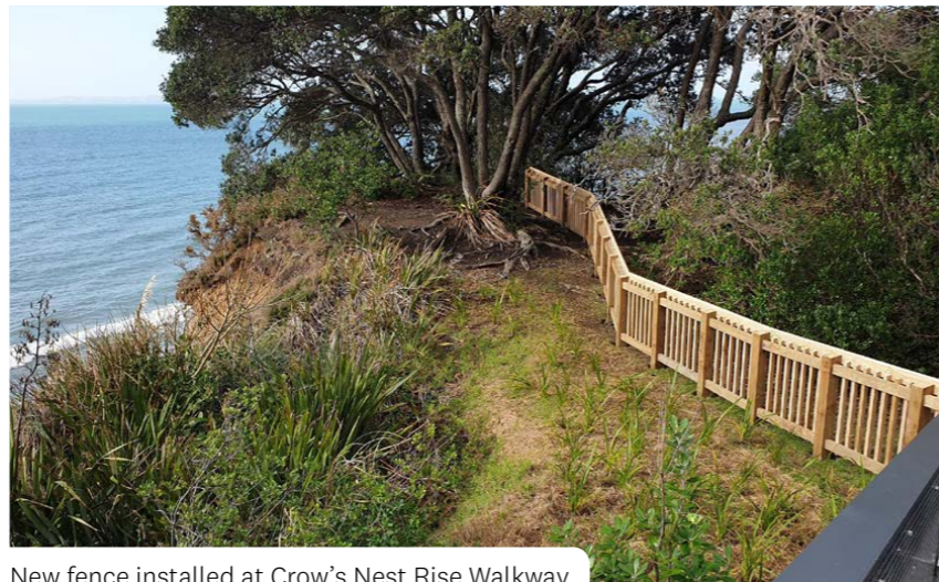
New fence installed at Crow's Nest Rise Walkway
