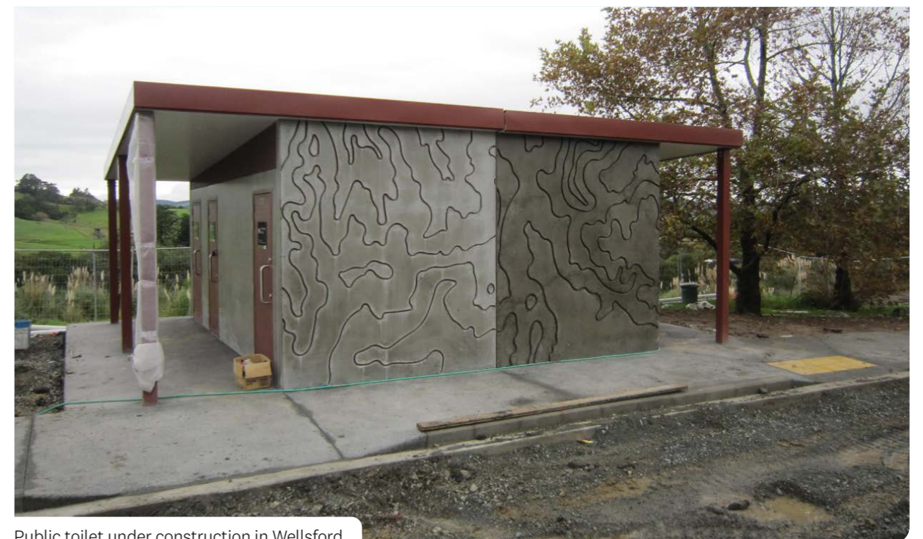
Public toilet under construction in Wellsford.
