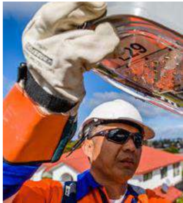
One of Auckland's 16,494 LED street lights is installed
