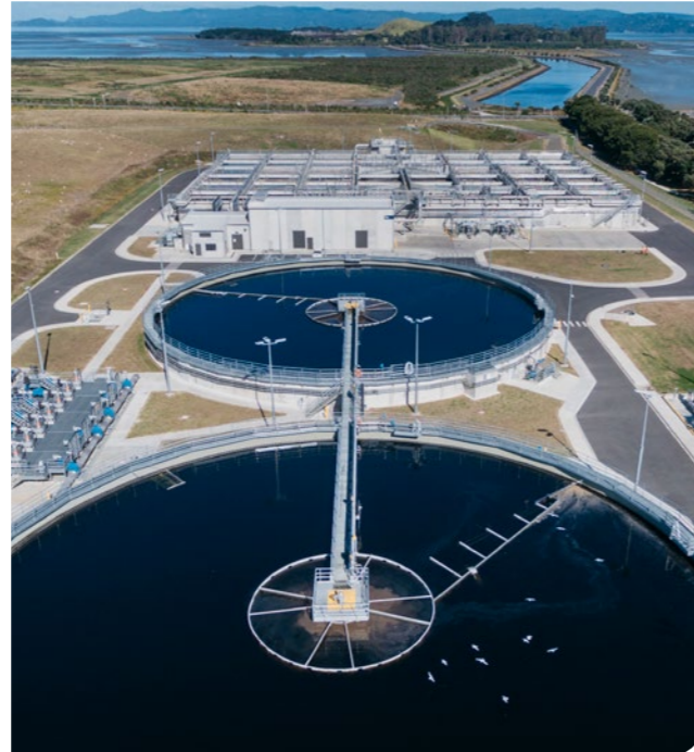
Māngere Wastewater Treatment Plant ▶
