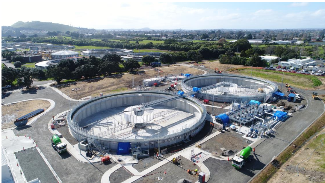
A bird's eye view of the BNR during construction.
