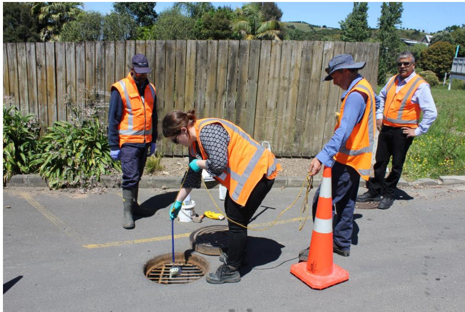
Inflow and Infiltration team investigating a manhole.
