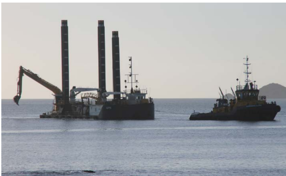
Tug pulling a barge into Tiri Channel to pick up the Army Bay tunnel boring machine
