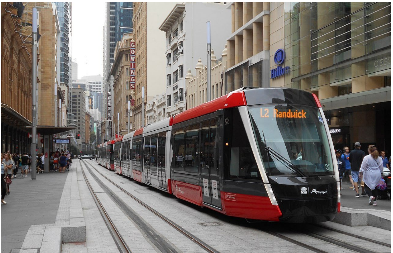
Figure 2: George Street in Sydney's City Centre, where space previously used for traffic lanes has been reallocated to create a light rail corridor and wider footpaths 3
