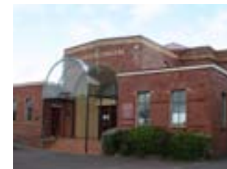
Connect to heritage building
