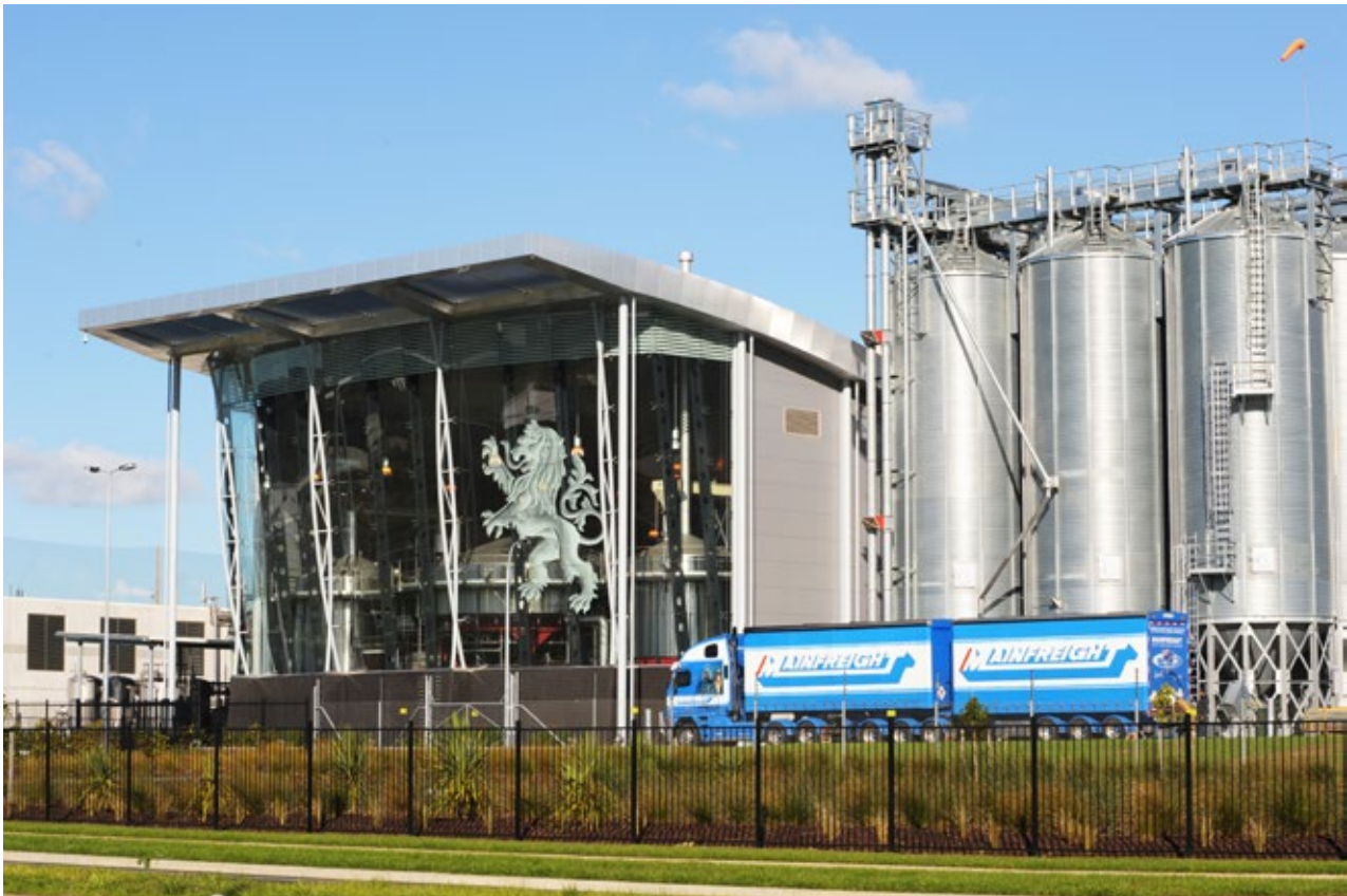
Lion have made East Tāmaki the home of their state-of-the-art brewery and beverage manufacturing and warehousing facility. Credit: Greater East Tāmaki Business Association.
