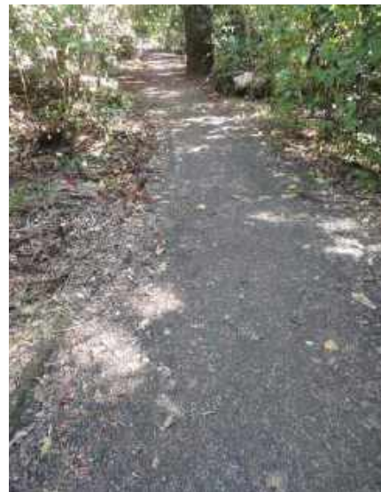
Basalt chip compacted aggregate tracks Use in forest areas
