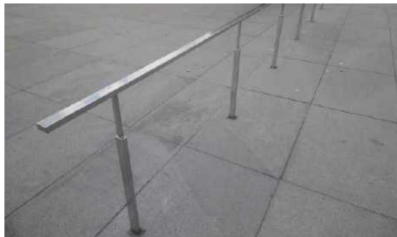
Custom stainless steel handrail - use in Museum surrounds To match existing
