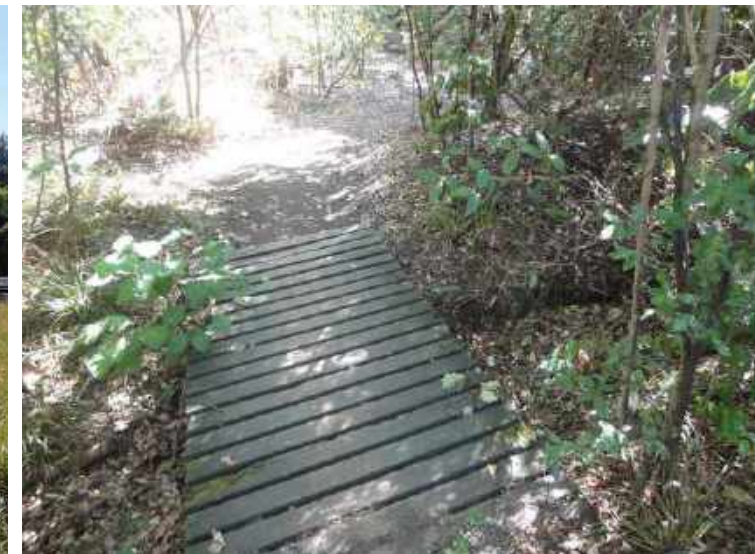
Timber boardwalk Use in forest areas over drainage flows, tree roots or flood plains
