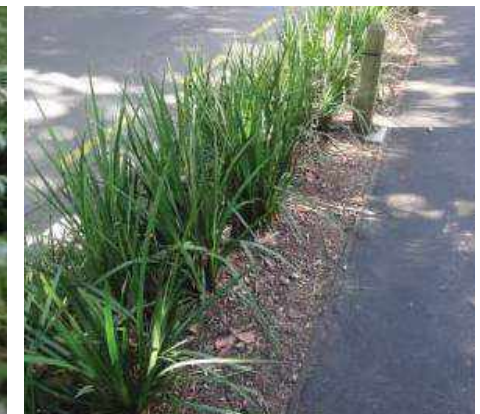
Use planting to separate vehicles from pedestrians and as a stormwater device.
