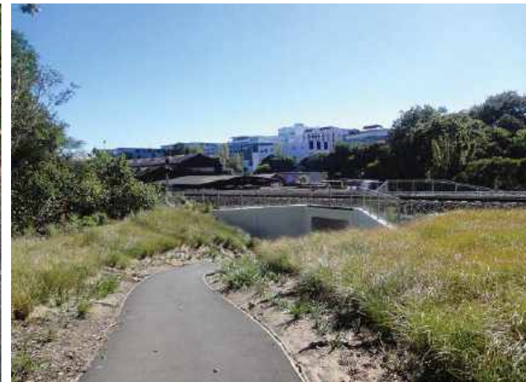
Asphalt paths with timber edging Use in forest areas where a high level of accessibility is required
