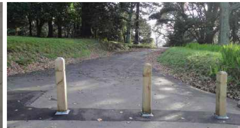
700mm x 150mm x 150mm H4 pine bollard - use in forest areas Notes: include chamfered top and notch groove
