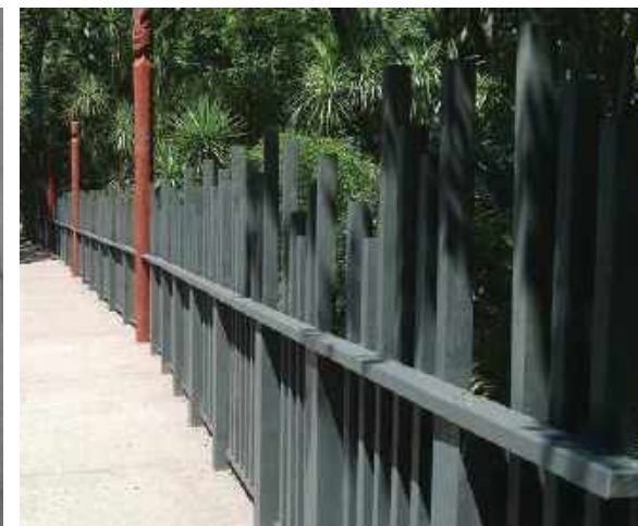
Custom timber palisade fence - use in forest areas Notes: pou to be carved by selected iwi artist
