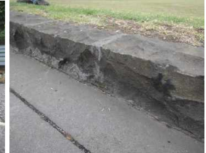
Basalt kerbstones - for use wherever kerbs are required Reuse existing stockpiles of kerbstones where possible
