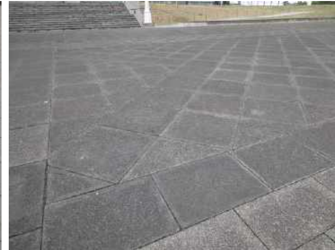
Concrete pavers - for use on Cenotaph consecrated ground To match existing - for renewals only
