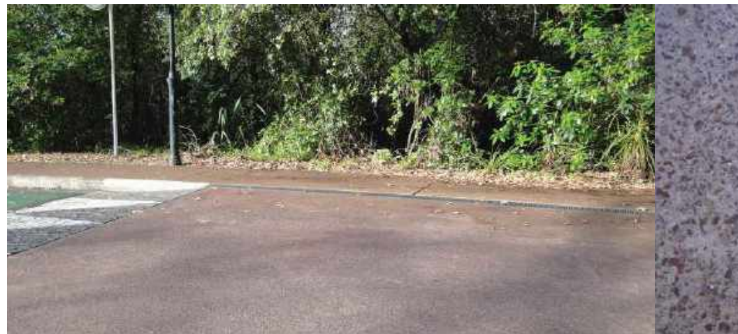
McCallums red chip exposed aggregate concrete Use for paths along roads and/or are not historic. Not for use in bush tracks or around Museum.
