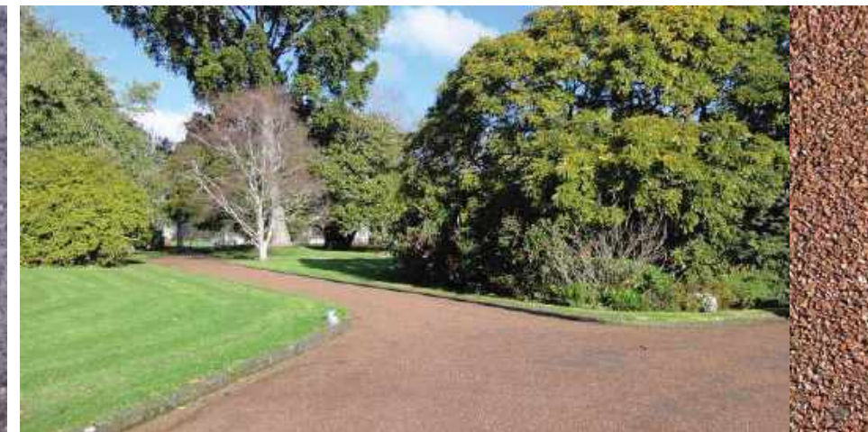
McCallums red chip sealed asphalt Use for paths along roads or that are historic. Not for use in bush tracks or around Museum.
