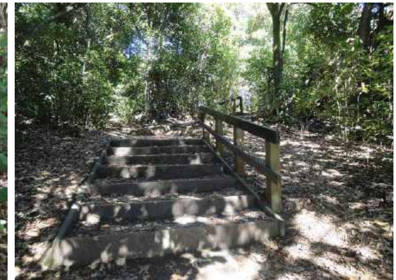
Timber boxed steps with basalt aggregate (timber handrail if required) Use in forest areas to traverse steep gradients
