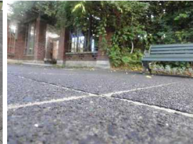
Concrete pavers - for use at Wintergardens To match existing - for renewals only
