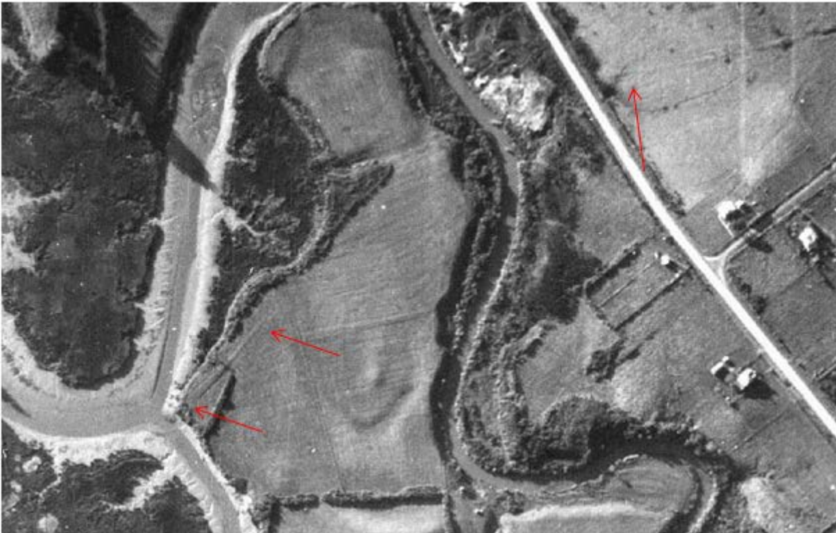
Figure 15. Traces of the 1859-64 tramway to the wharf at Abraham's Point are visible on this 1942 aerial photograph. The linear feature recorded as a ditch appears to bisect and thus post-date the tramway embankment. Shadows indicate that the feature recorded as a bank has planting along it.
