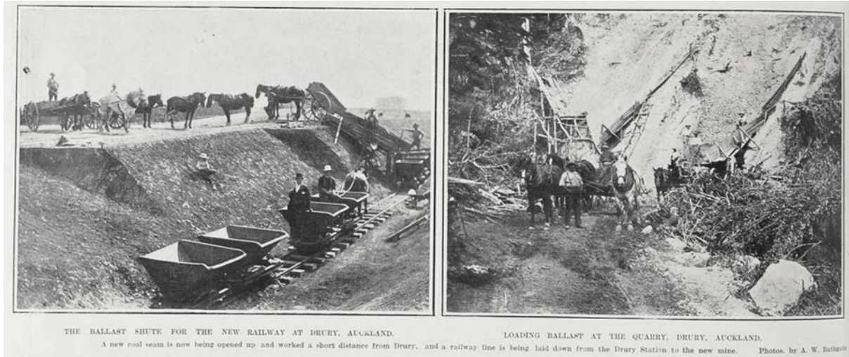
Figure 6. Transporting ballast material to construct the new railway line, 1905.
