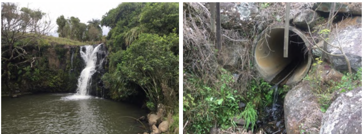
Figure 6: Representative photos of fish passage issues. A) a natural barrier to fish passage (large waterfall) and B) artificial barrier to fish passage (perched culvert).
