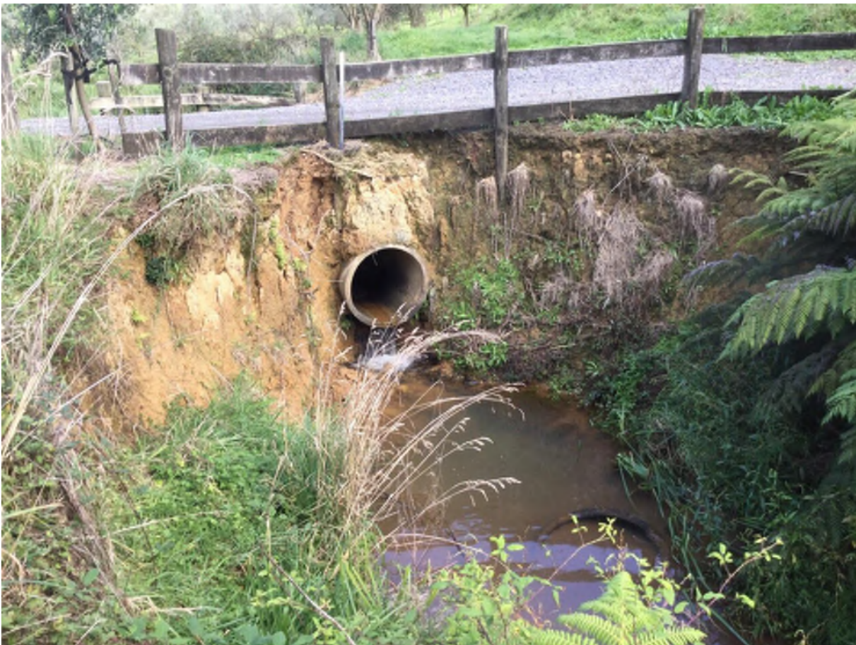
Figure 9: Significant erosion, and a fish barrier, associated with a rural, private asset.
