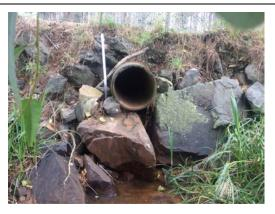
Perched culvert at downstream end of EO
