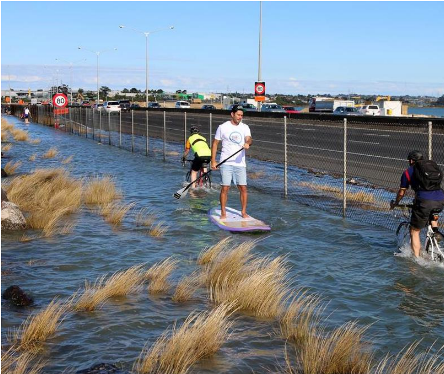
Figure 3: Inundation of State Highway 16 3
