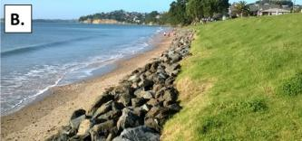
Figure 6-3: Photographs of coastal stretch 3 showing A) Red Beach Surf Club and B) supporting revetment (facing south)
