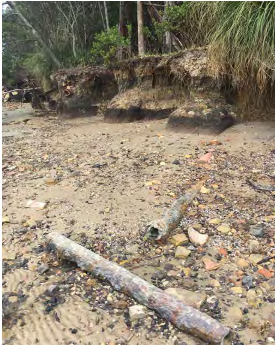
Remnants of iron and ceramic pipes along the foreshore, the iron pipes have rusted and the ceramic pipes have broken
