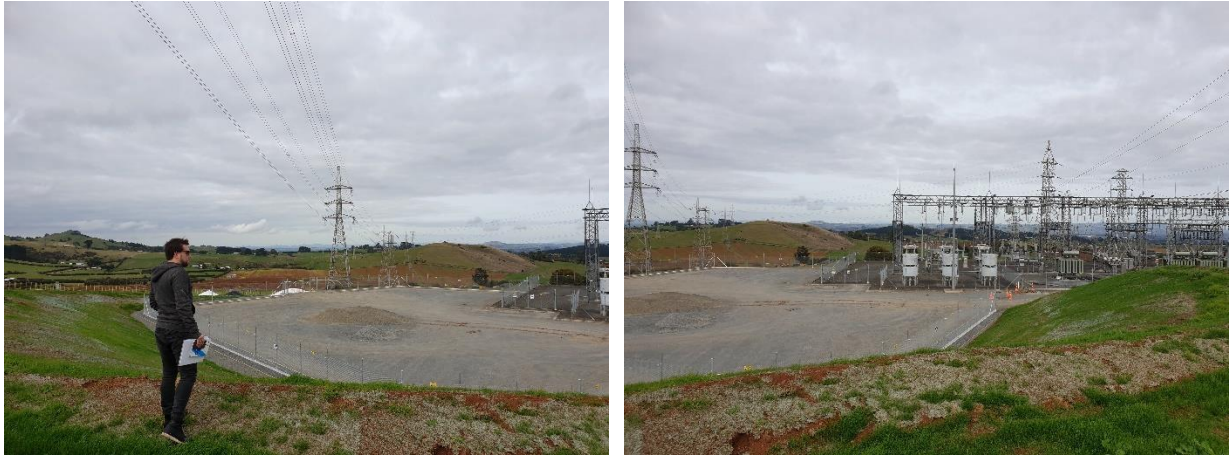
Photo 1 and 2: Platform created by enabling works (taken May 2021)
