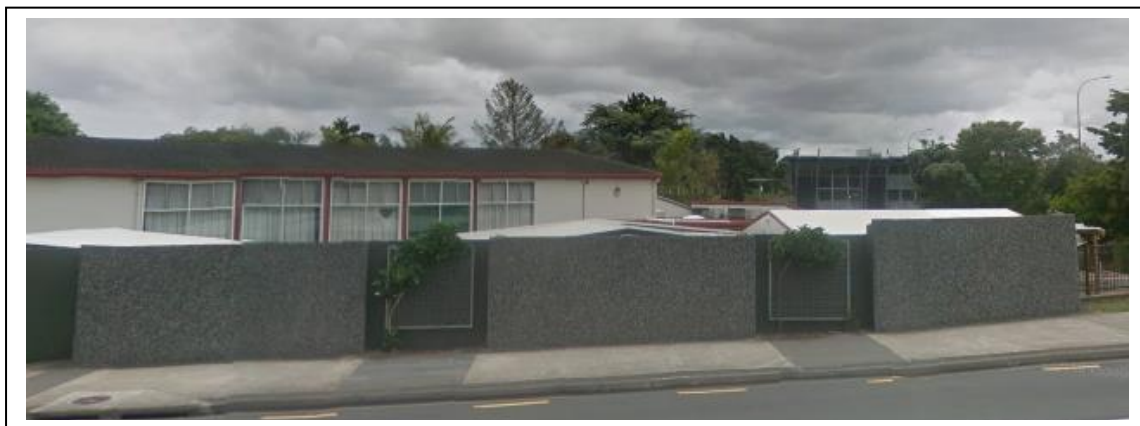
Figure 6: Two Landscape Bays to be Removed
