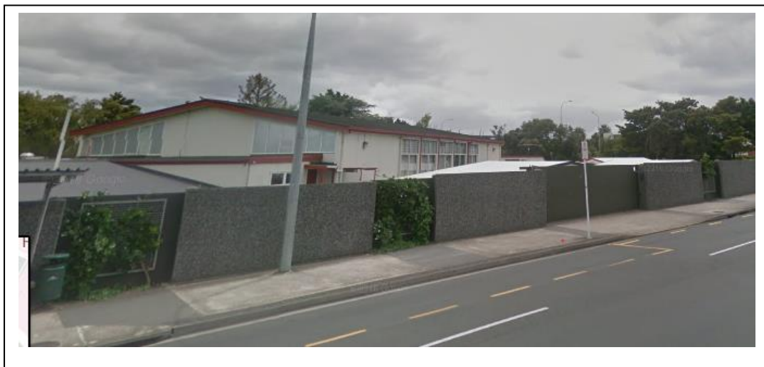
Figure 4: Acoustic Fence with Sliding Gate, with old school hall behind
