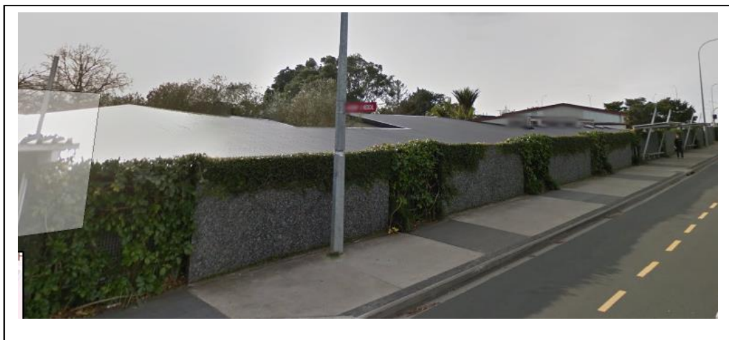
Figure 3: Acoustic wall with landscaping, looking east toward Wairua Road (Source Google Maps)
