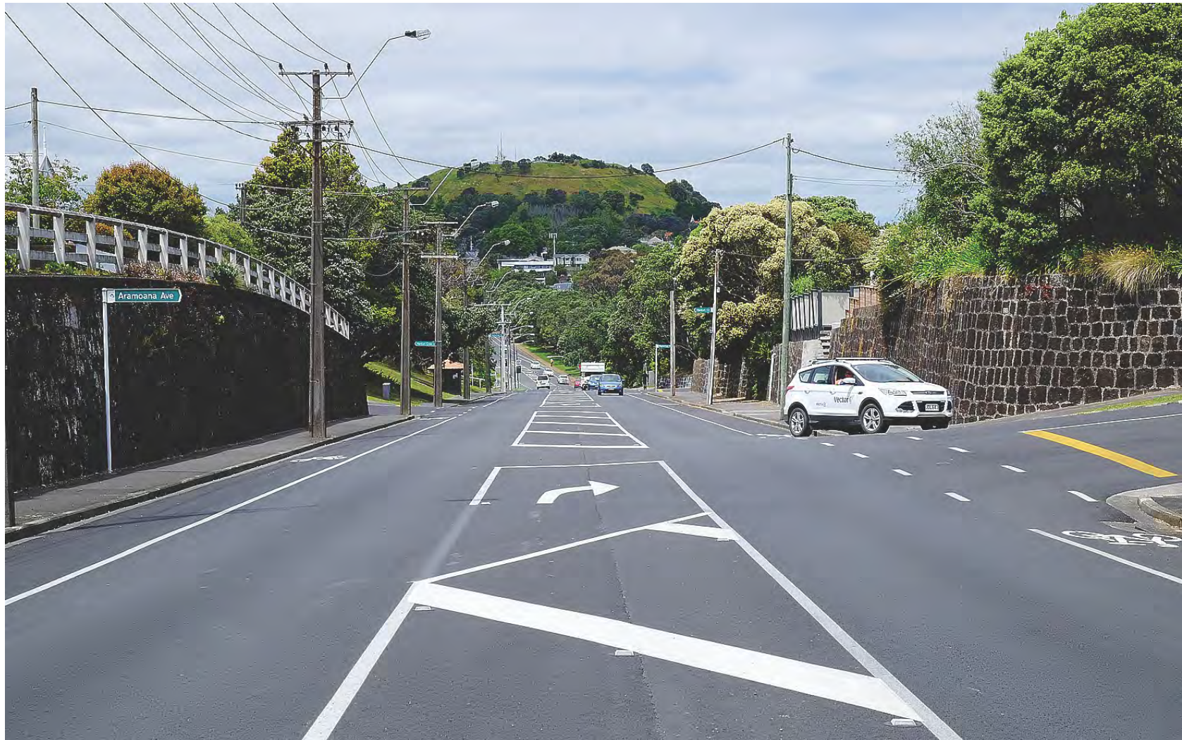
View V03: Photo 1 of 1 The Individual Cone (60mm lens equivalent) (This photograph is indicative only; field based analysis is required for assessment purposes)
