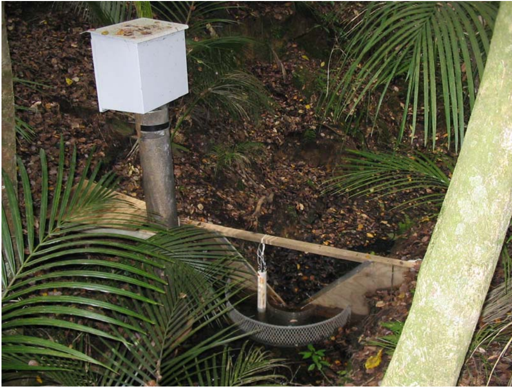
Figure 8: Bush weir and sonde.
