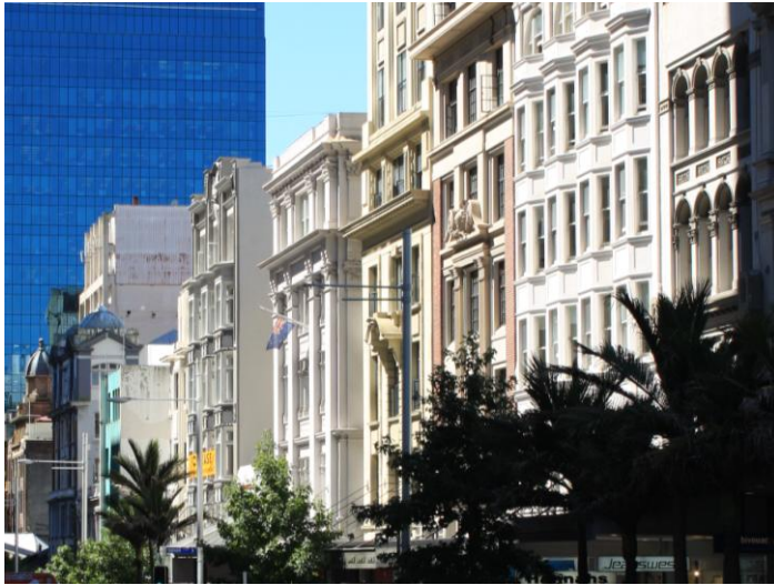
Fig 7: Showing a group of buildings on the eastern side of lower Queen Street with strong character (with the Deloitte Building in the background).
