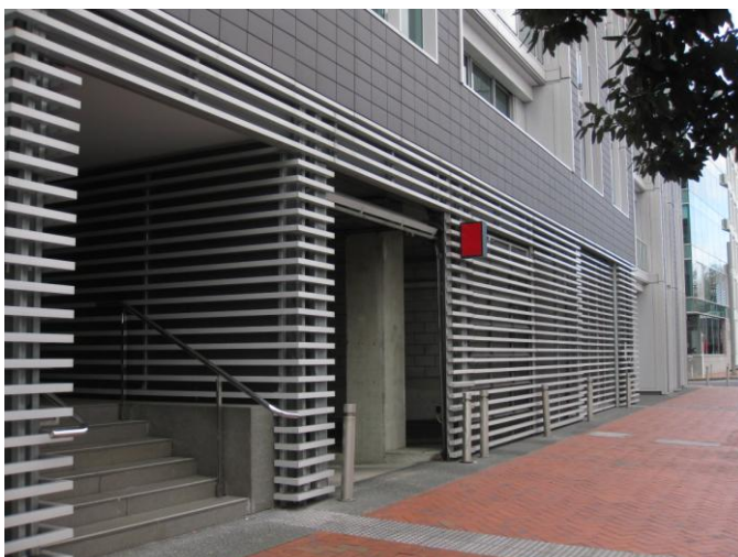
Fig 38: showing the eastern façade of the Westin Hotel on Viaduct Harbour Ave.
