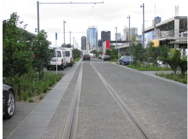
Fig 47: showing Jellicoe Street after the recent upgrade.
