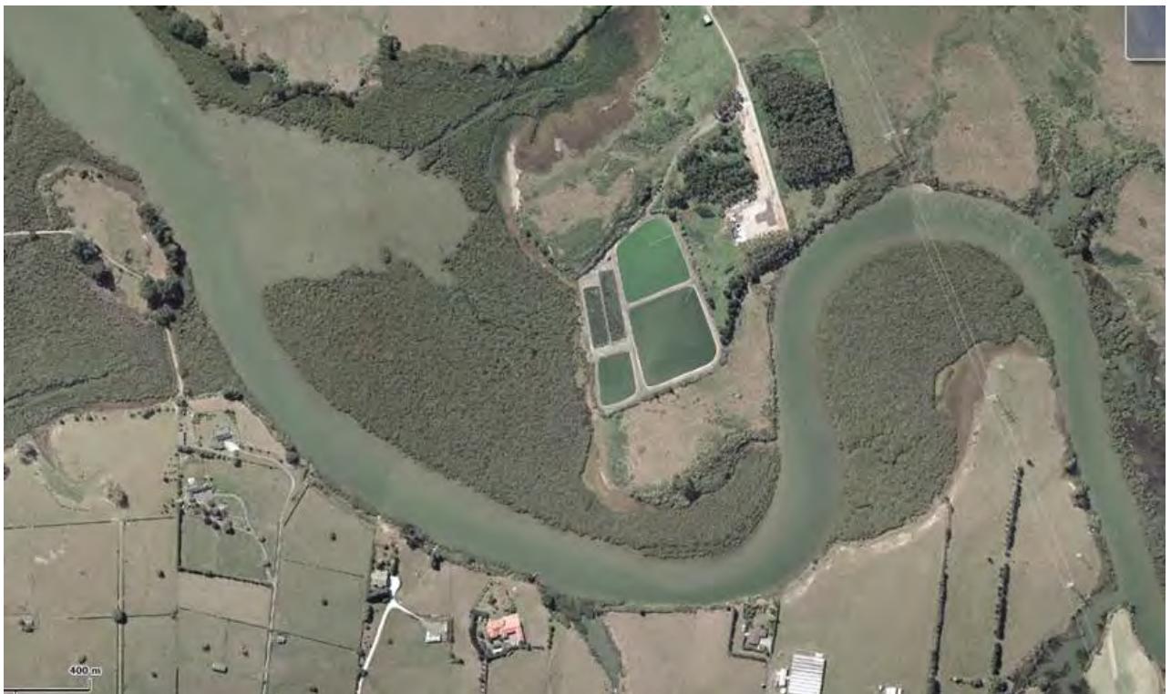
Figure 6-3: Aerial image of Drury WWTP (2006)
