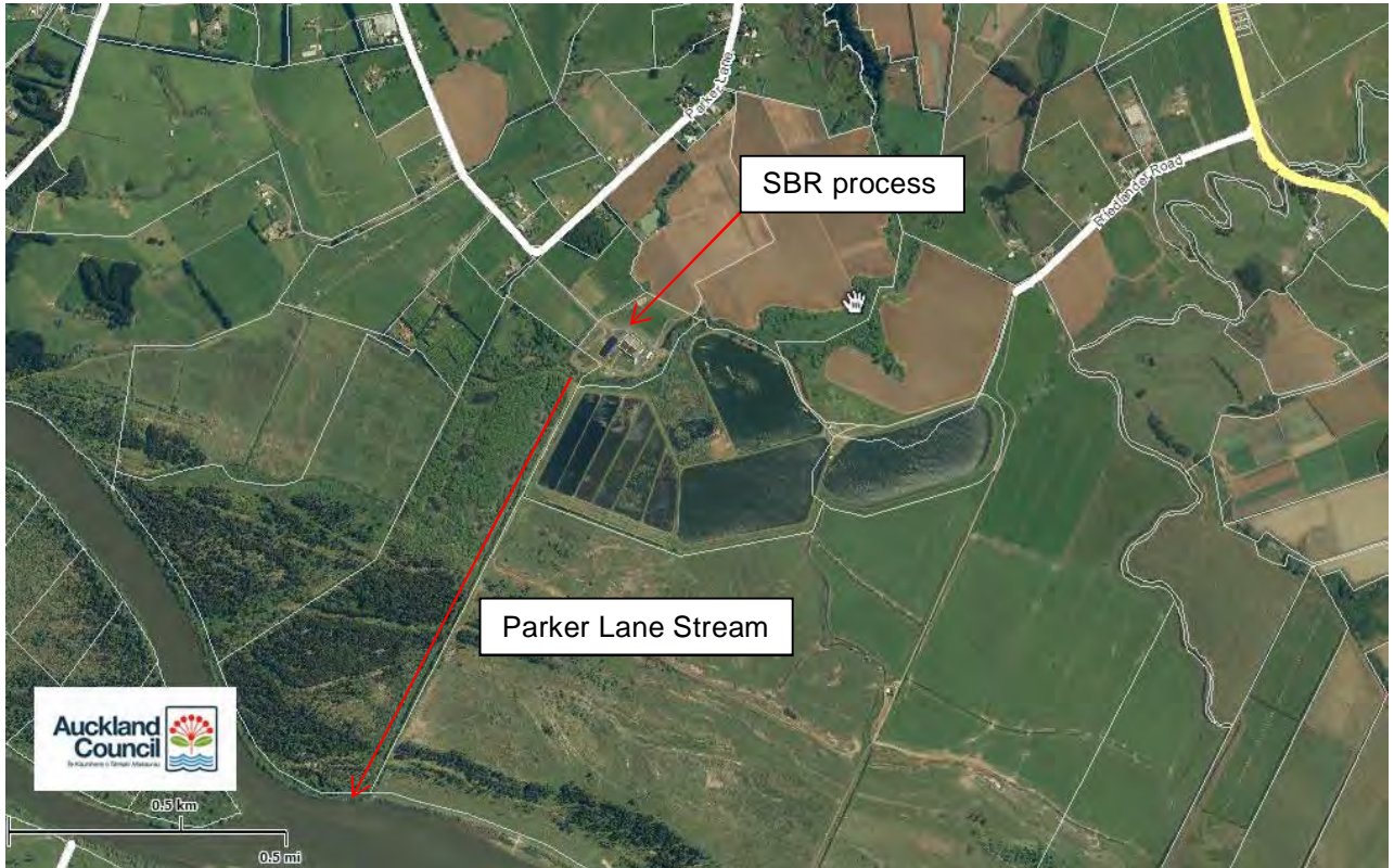
Figure 6-2: Pukekohe WWTP site
