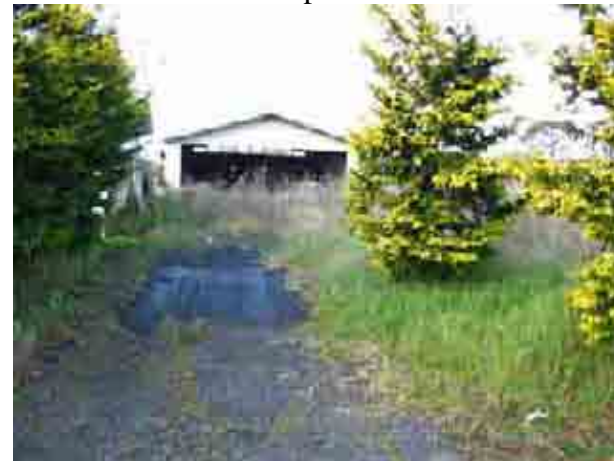
Photo 8. Shed/garage building at 1249 Paerata Road.
