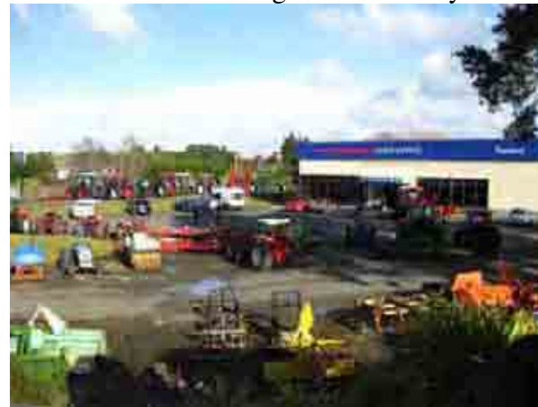
Photo 4. View south to the main building from the storage yards along Heights Road.
