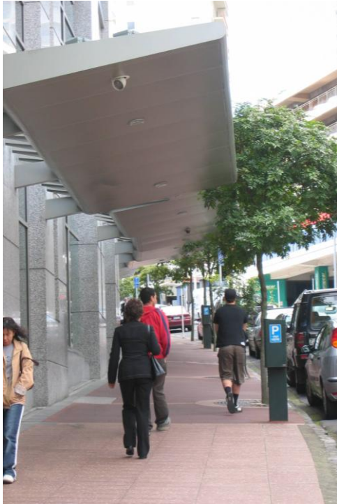
Fig 39: looking east on Shortland Street
