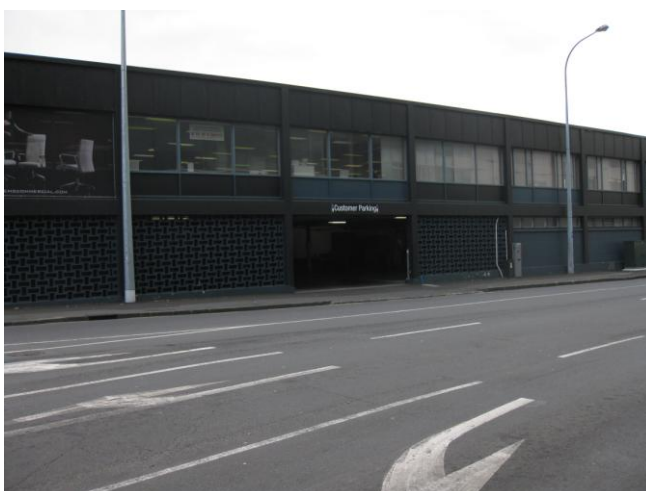
Fig 27: a building with a ground level frontage that is devoid of activity negatively affects a person's perception of safety when walking in the street.
