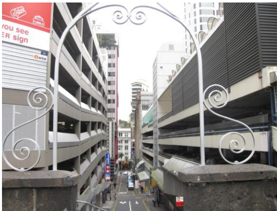
Fig 22: showing two carparking buildings and poor street interface on Durham Lane.
