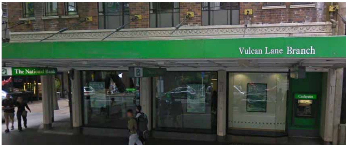
118 Queen Street, corner of Vulcan Lane
