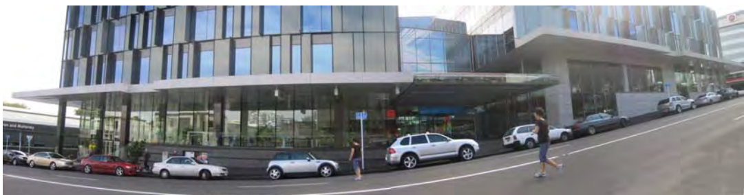
Telecom building (167 Victoria Street West)
