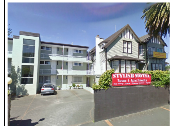
5. This motel comprises of two buildings that are from two different eras. The newer building has looked to fit in with the original building by mimicking colour, and by building to the same height. It would be more successful if it had included a little more detail and parking was at the rear.
