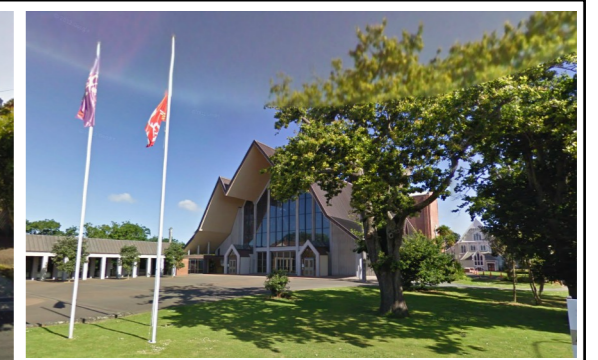
2. This cathedral is located across the road from the site. It is a grand structure that has strong cultural importance in the region. It is a large, high building with strong forms that is clad in a mixture of materials including brick. It has been set back from the street to emphasize its importance.
