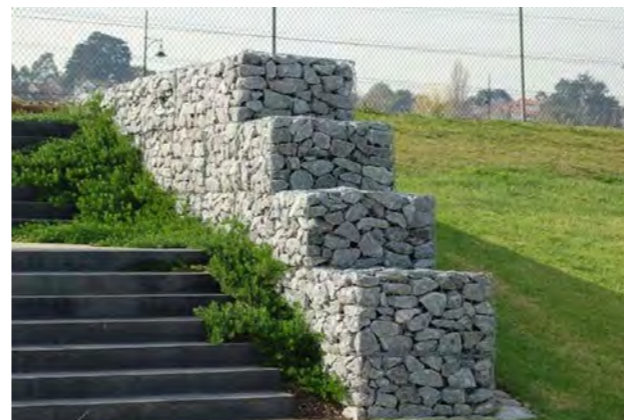
Walls using stone filled gabion mesh baskets
