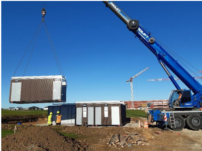
Photo: Installation of the toilet and changing facility, June 2023
